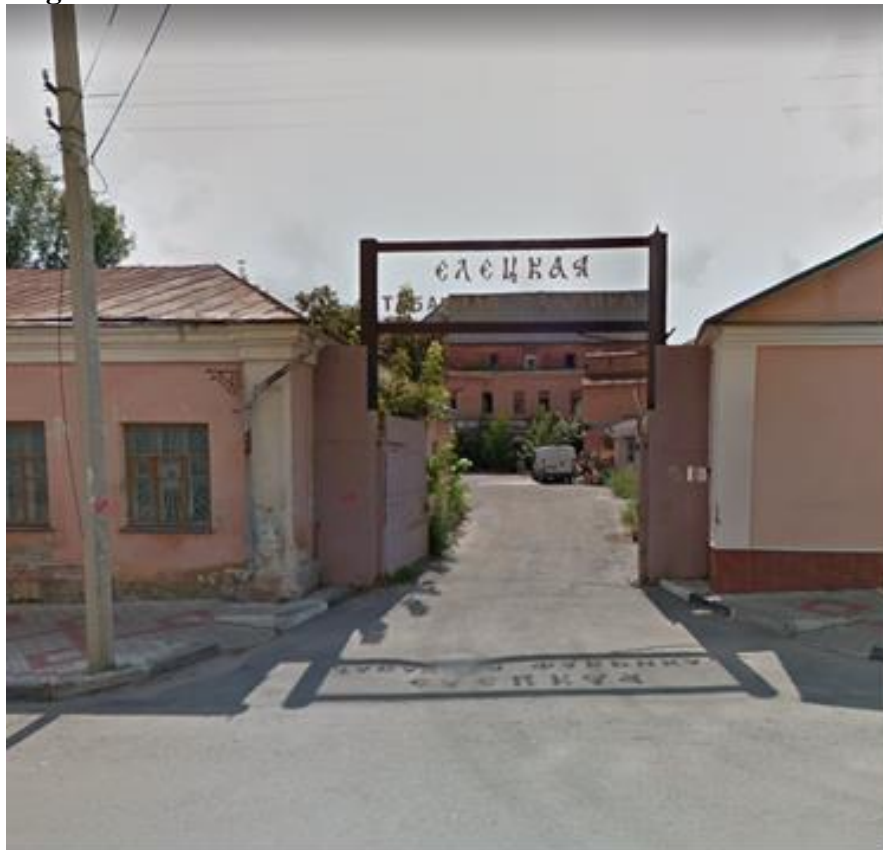
Photo of the gate
