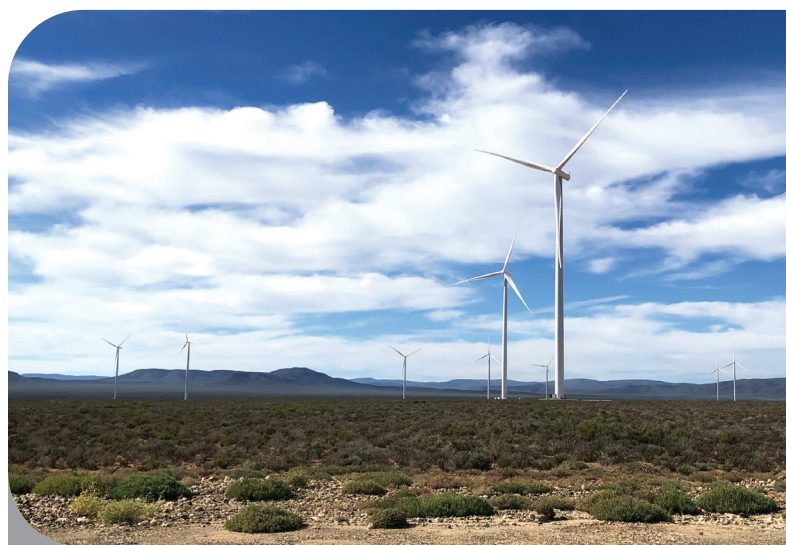
Onshore Wind Farm financed by the project, South Africa
